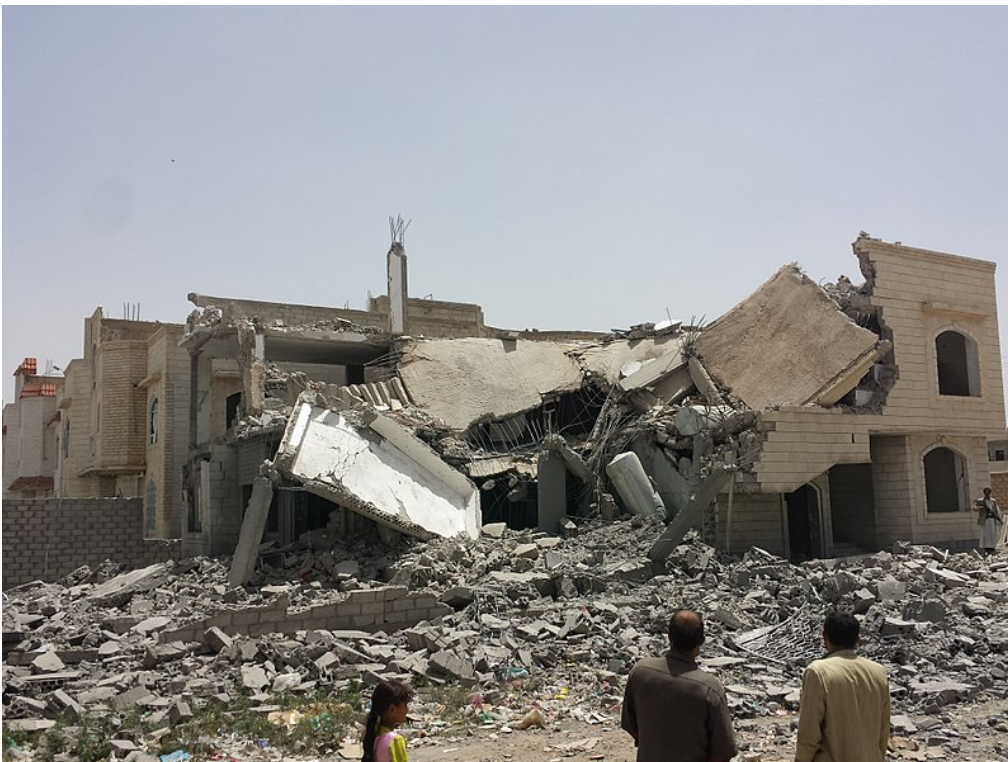
Destroyed house in the south of Sanaa, 13 June 2015 (Source: Wikimedia Commons )
