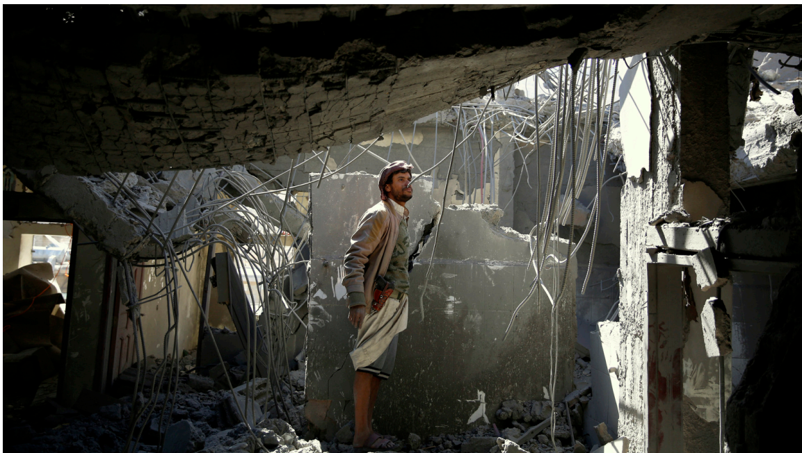
A man inspects his home destroyed by airstrikes in Sanaa, Yemen, Monday, Jan. 4, 2016. (AP/Hani Mohammed)
