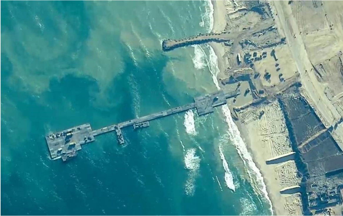
Overhead image of the connection of the Gaza Pier shortly after completion by US military forces on May 16, 2024 (From the Public Domain)
