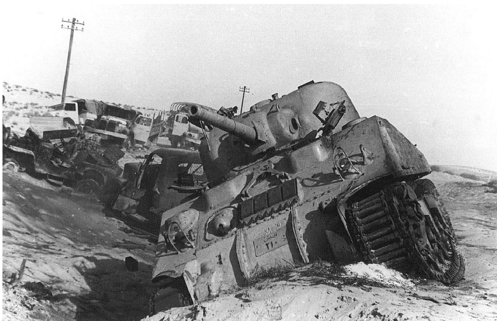
Damaged tank and vehicles, Sinai War, 1956. (Source: Public Domain)
