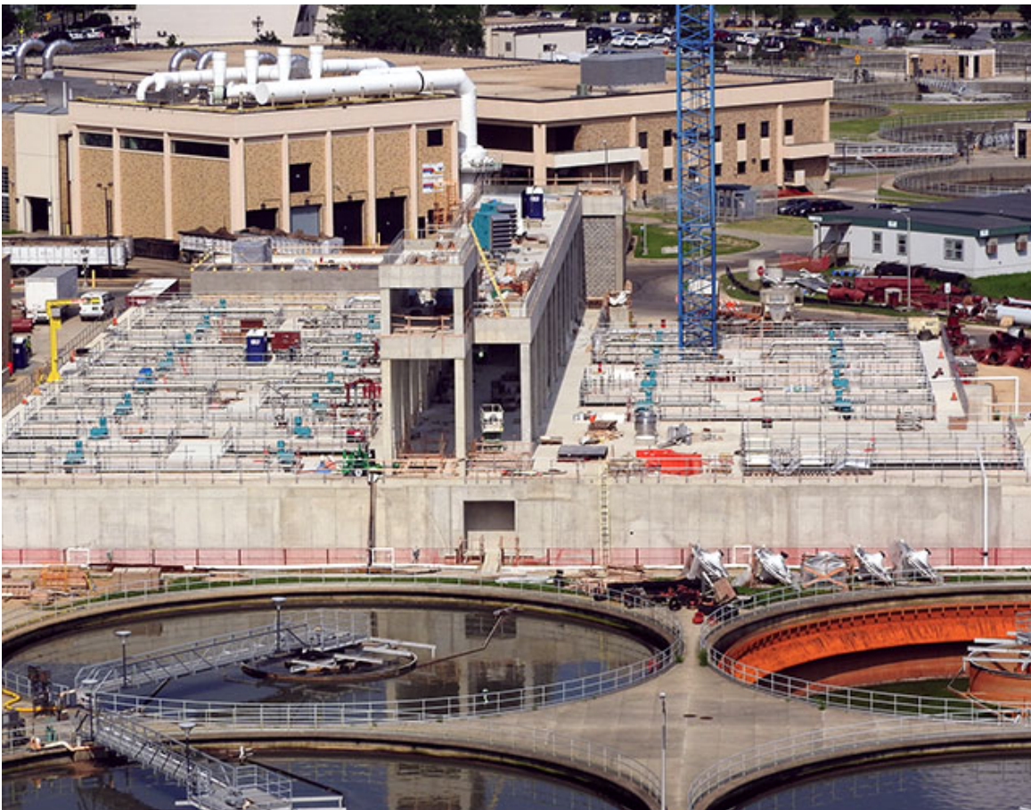
Filtrate treatment facility at Blue Plains. [Source: pconstruction.com ]
