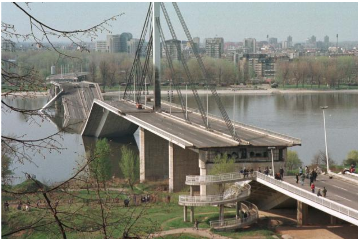
A bridge in Novi Sad (Tanjug, file)
