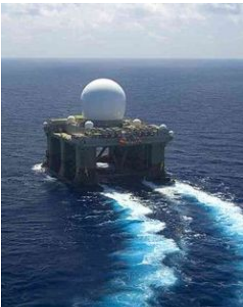
Sea-Based X-Band Radar, part of Ground-based Midcourse Defense system
