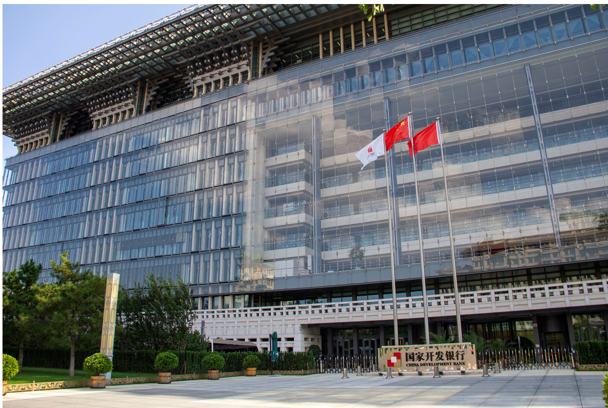
China Development Bank headquarters (Licensed under CC BY-SA 4.0)
