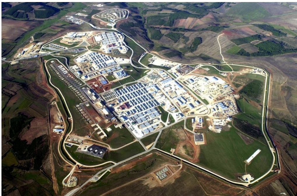
Aerial photo of Camp Bondsteel, KFOR, Task Force Falcon Public Affairs Office (Source: Wikimedia Commons )
