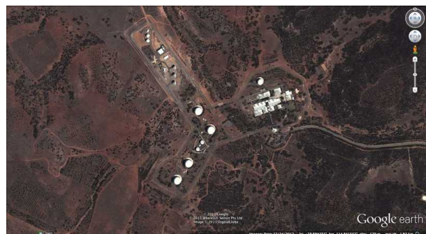
Australian Defence Satellite Communications Ground Station, Kojarena. Google Earth, December 2012. MUOS and WGS ground terminals are located in the upper left arm of the facility
