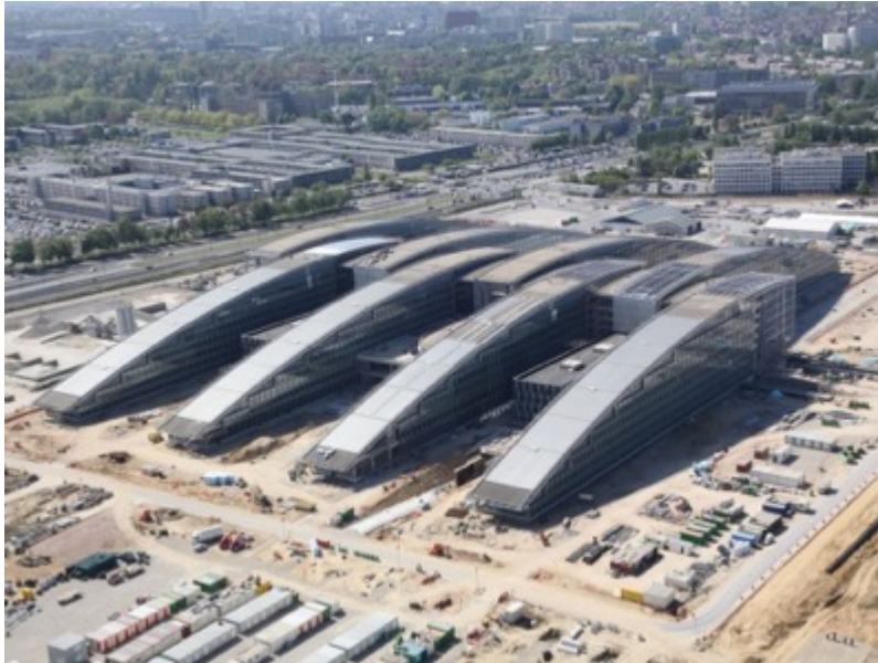
The new headquarters of the Alliance, in Brussels, has just been built for the modest sum of one billion dollars.
