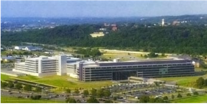
Defense Intelligence Agency headquarters, Bolling Air Force Base, Washington DC (Source: Wikimedia Commons)
