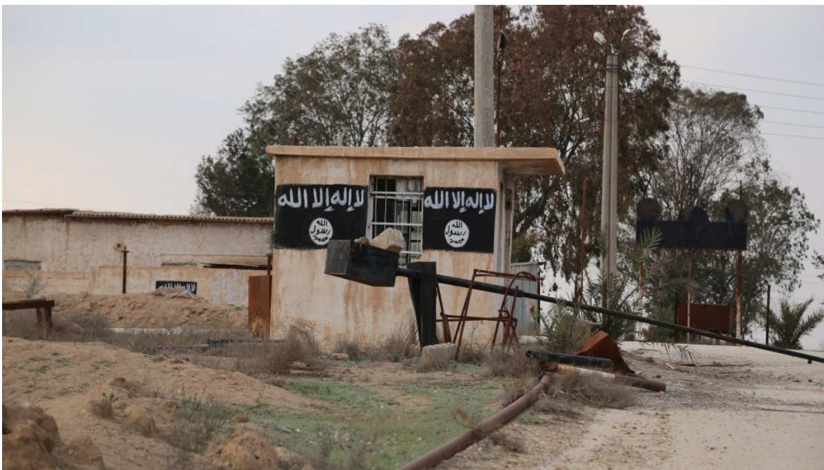
One of the buildings used earlier by Daesh (source: RT)
