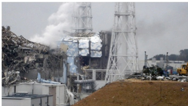
Damaged reactors at Fukushima Daiichi
