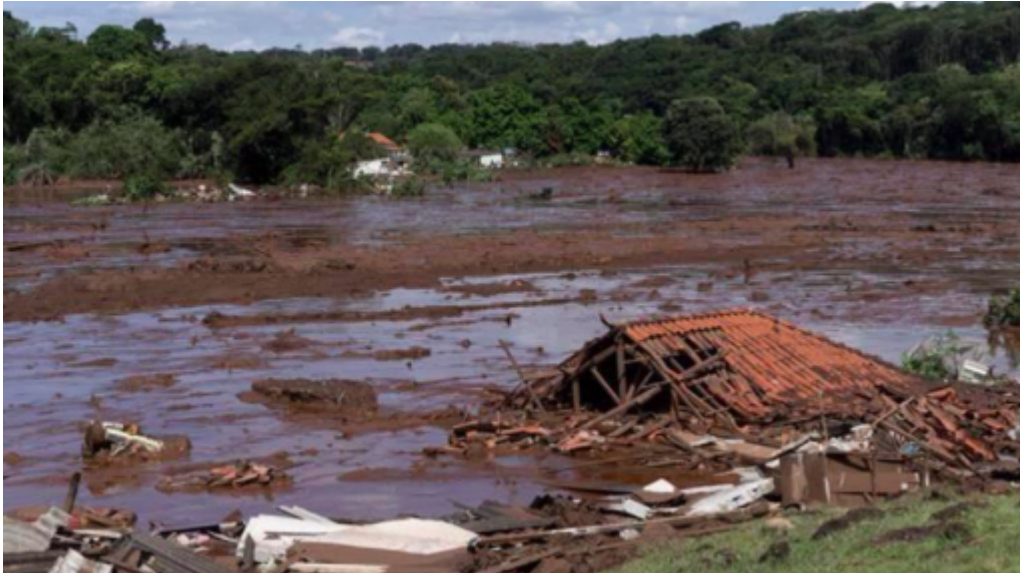
A demolished home lies in ruins after a dam collapsed near Brumadinho, Brazil the day after the dam failure
