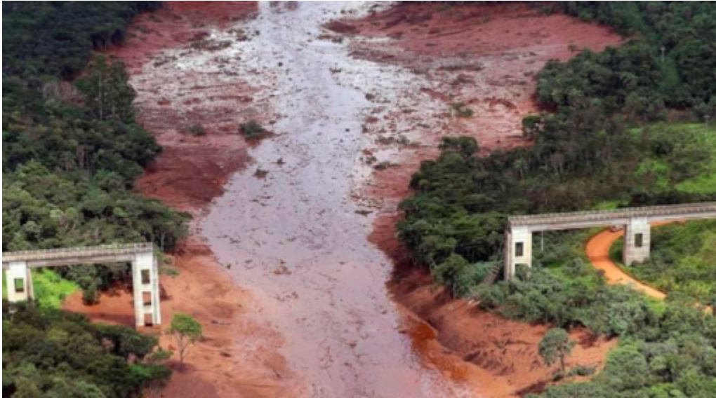
An aerial view shows a destroyed bridge after a dam collapsed in Brumadinho, Brazil
