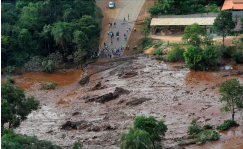
Totally washed-out highway that may have once crossed a small river
