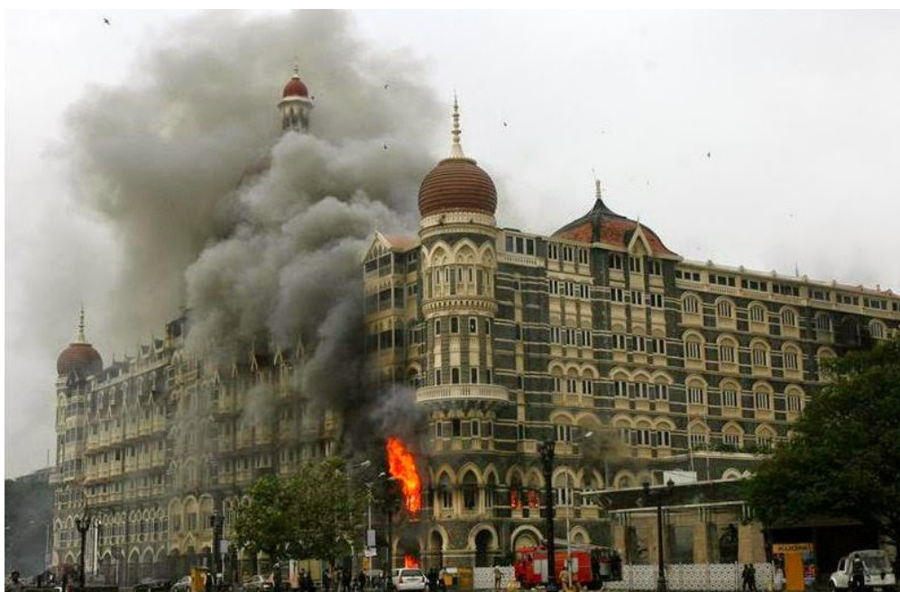
The Taj Mahal Hotel burning after the terrorist attacks in Mumbai (Source: Haunted India)
