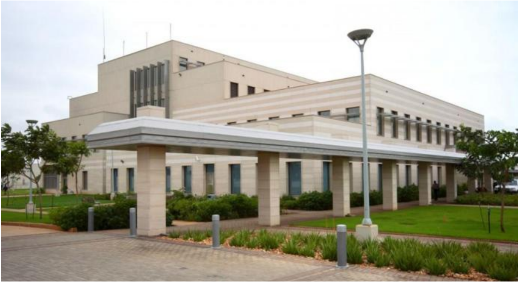
U.S. embassy compound in Lusaka. [Source: bilharbert.com ]
