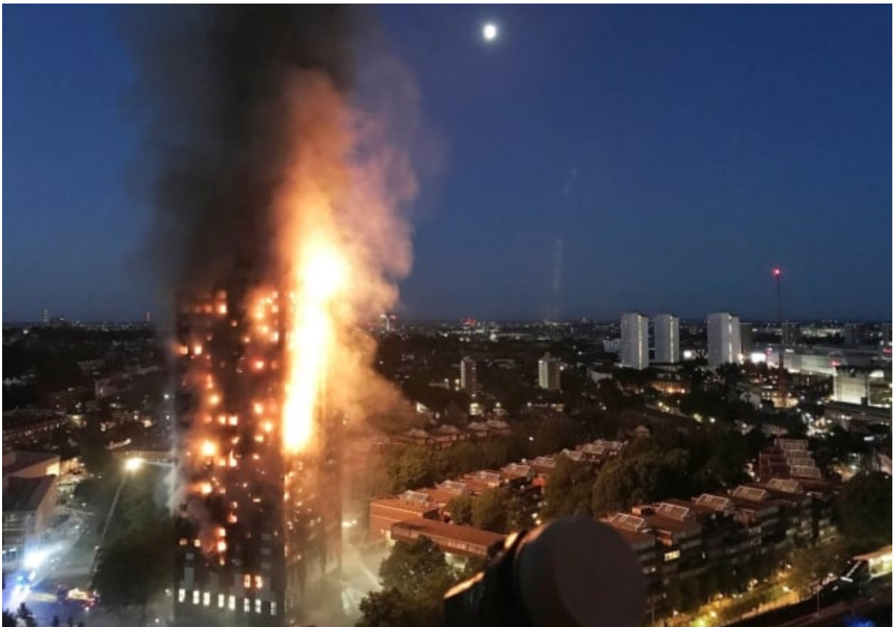
Grenfell Tower on fire. Source The New European
