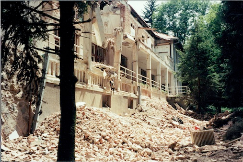
Rear of nursing home in Surdulica. Photo: Gregory Elich.
