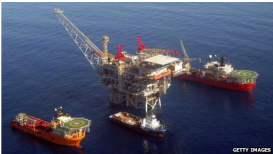
| The Tamar drilling platform sits 25km off the coast of Israel
