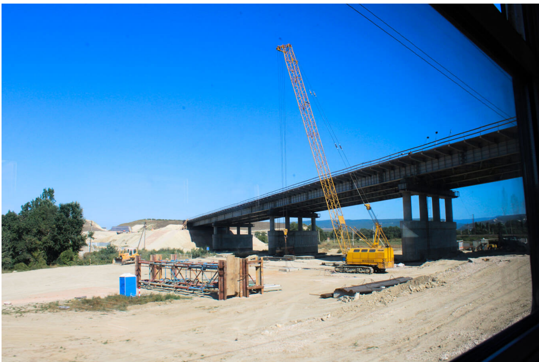
Construction dots the train ride to Sevastopol. Photo | Eva Bartlett
