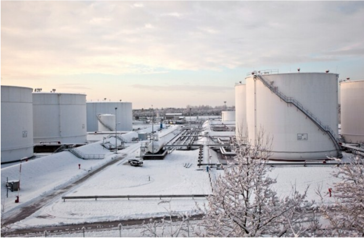
Oil storage tanks in Russia. [Source: energyintel.com ]
