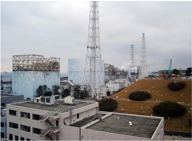
In some of the reactors – especially those to the right of the photo – the area in which the spent fuel pools are located appears to be severely damaged.
