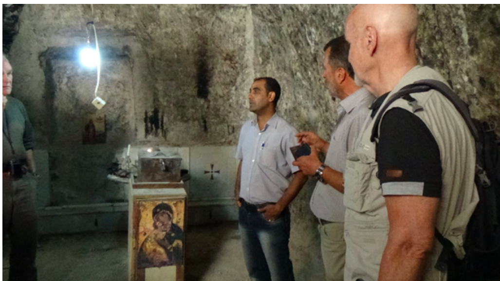
Mark Taliano, September 2016. Terrorist-damage (FSA, al Nusra Front) to the Shrine of Saint Takla, Maaloula, Syria.
