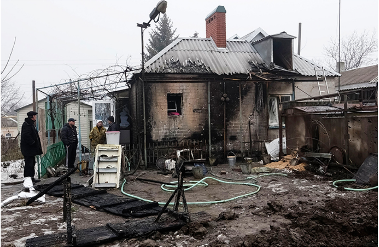
Local residents inspect their home, which was damaged by shelling in the village of Sartan, near Mariupol (Reuters / Nikolay Ryabchenko)
