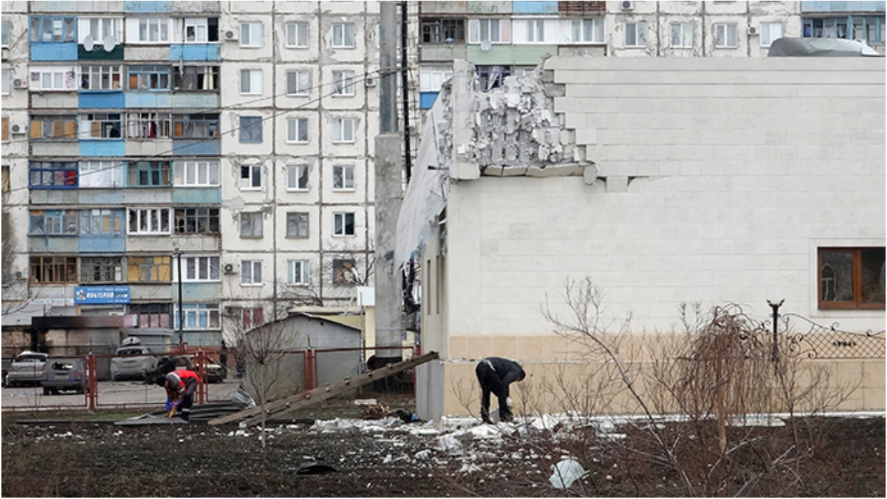
People remove debris near the building damaged by shelling on Saturday in Mariupol, eastern Ukraine, January 25, 2015 (Reuters / Nikolay Ryabchenko)
