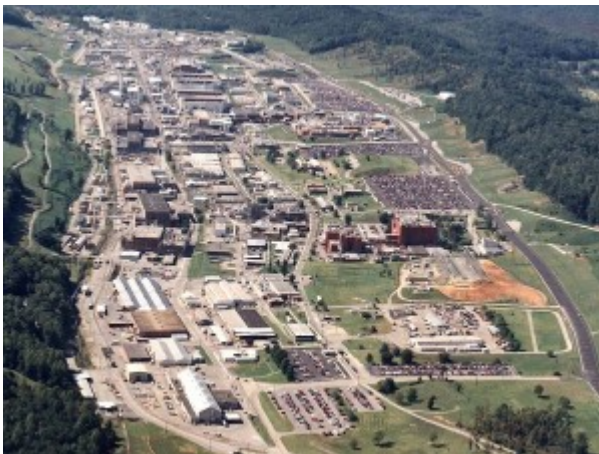
Oak Ridge nuclear plant in Tennessee.
