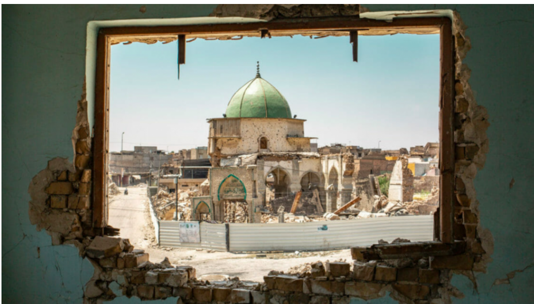
The Mosque of al-Nuri seen through a damaged window – West Mosul
