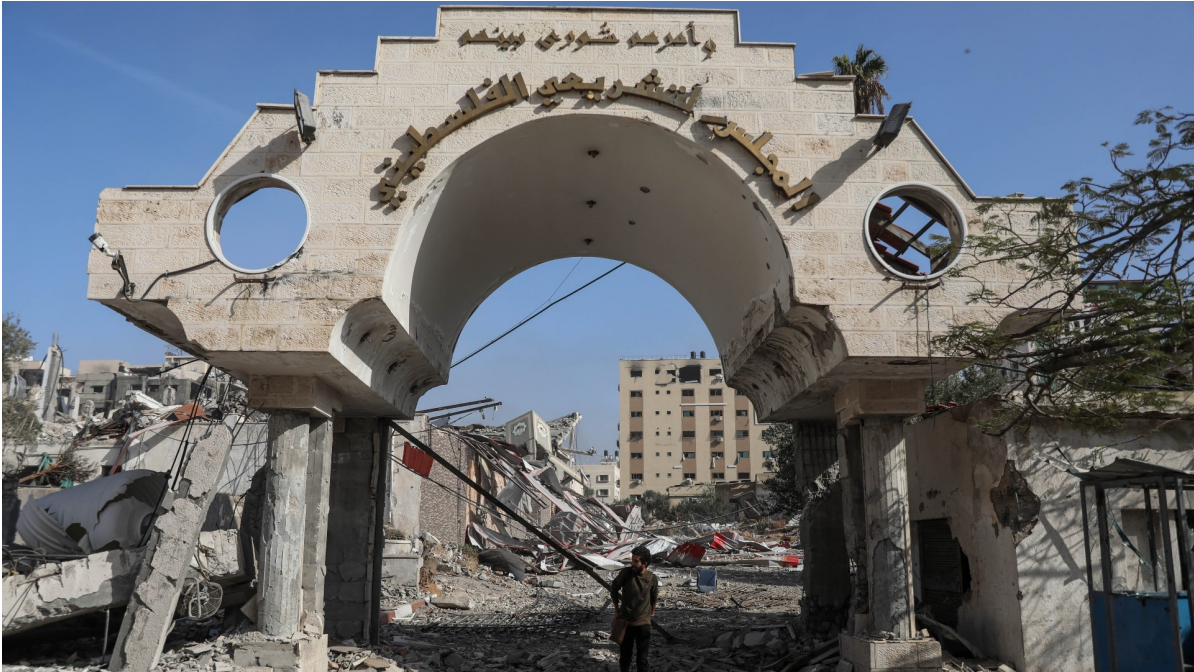
The gate of the damaged headquarters of the Palestinian legislative council in Gaza pictured on 24 November 2023, following intensive Israeli air strikes on the northern Gaza Strip (MEE/Mohammed al-Hajjar)
