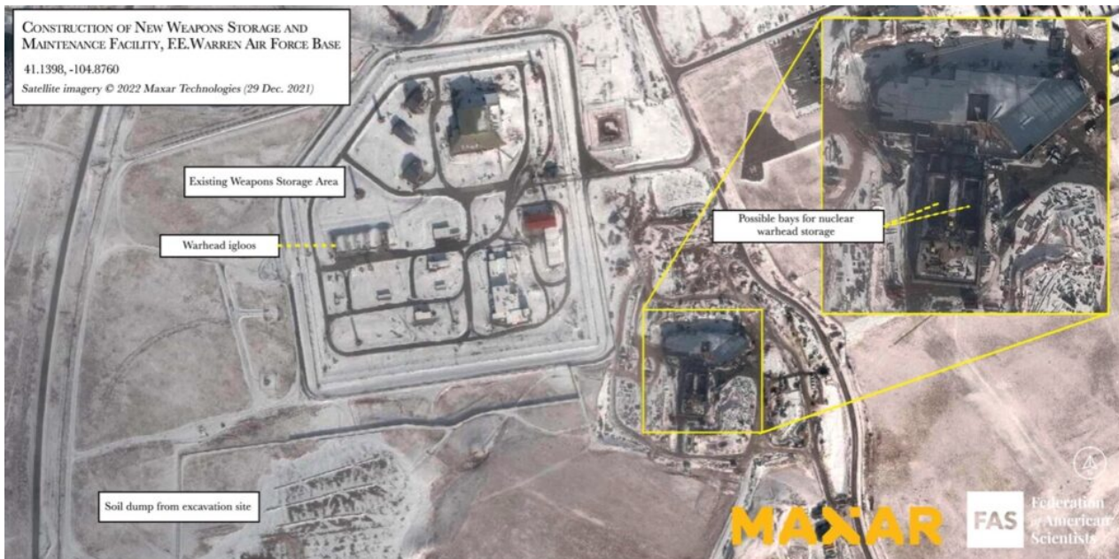
Figure 2: A new underground nuclear weapons storage facility is under construction at F.E. Warren AFB for storage of W78 and W87 warheads for Minuteman III ICBMs. Image: © 2022 Maxar Technologies.
