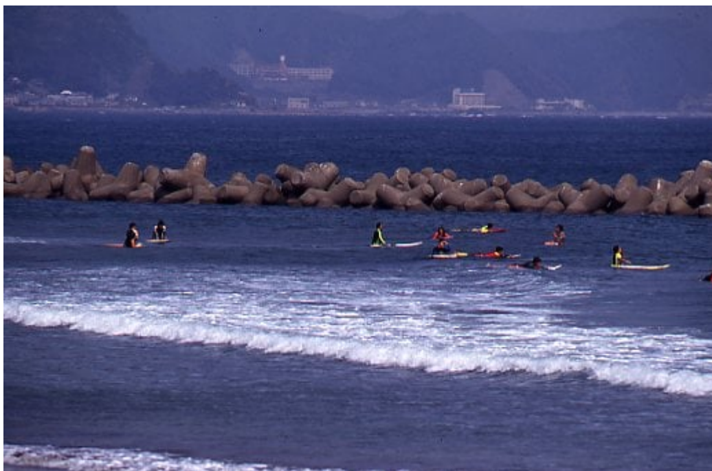
The giant sea walls of concrete tetrapods used off the eastern coast of Japan to protect smaller sea ports and fishing villages from waves. Photo c. Keith Harmon Snow,
