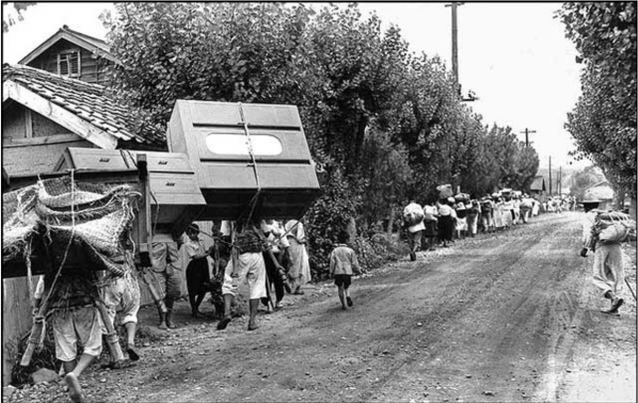
Long lines of refugees fleeing from Yongdong on 26 July 1950. The day before, hundreds of refugees were massacred by U.S. soldiers and warplanes at bridge at No Gun Ri, eight miles away.
