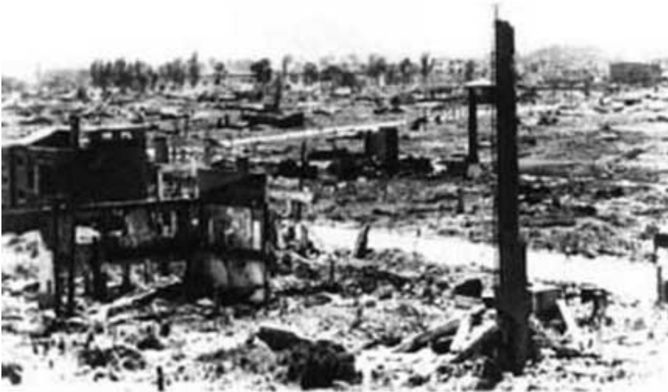
Pyongyang 1953. totally destroyed
