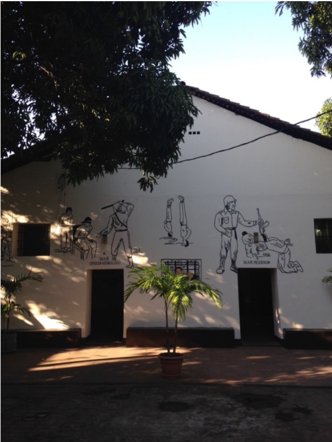
Former torture facility and prison run by Somoza's death squads in the city of León. [Source: Photo courtesy of Lauren Smith]
