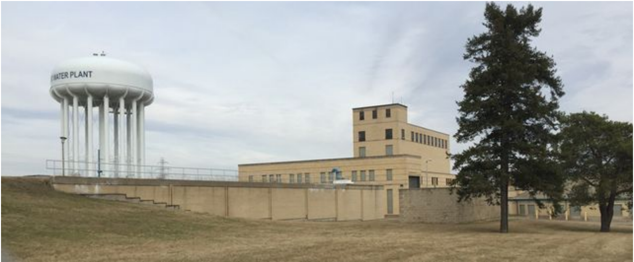
Image: The Flint water treatment plant
