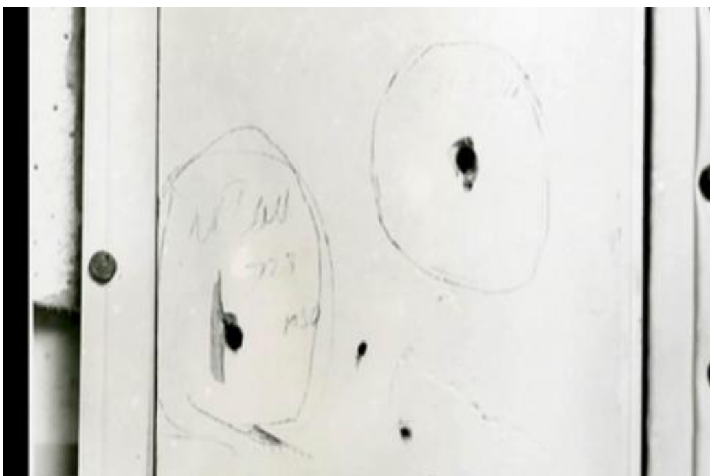
Marked bullet holes in doorframe. [Source: riversong.wordpress.com ]
