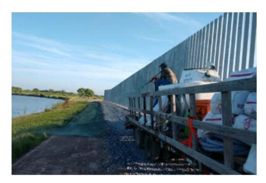
Fisher Industries has installed a 10-foot-wide road made with rocks to help address erosion issues while allowing access by Border Patrol agents. (Courtesy of Fisher Industries)
