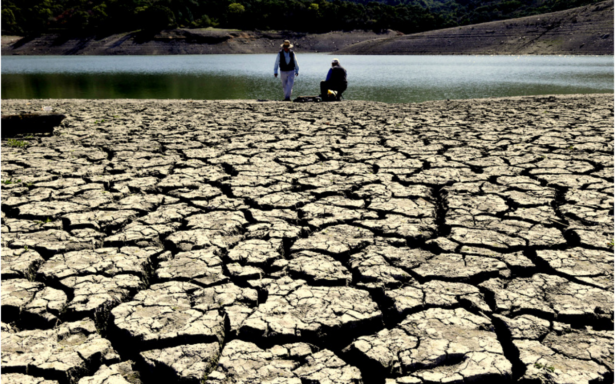
Cracks in the dry bed of the Stevens Creek Reservoir in Cupertino, Calif. Photo credit: Marcio Jose Sanchez/AP
