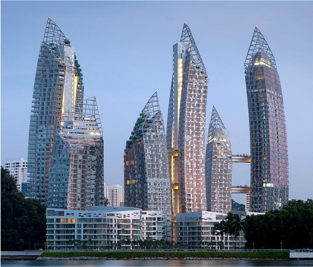
Reflections at Keppel Bay apartment complex in Keppel Bay, Singapore by Daniel Libeskind (2011)
