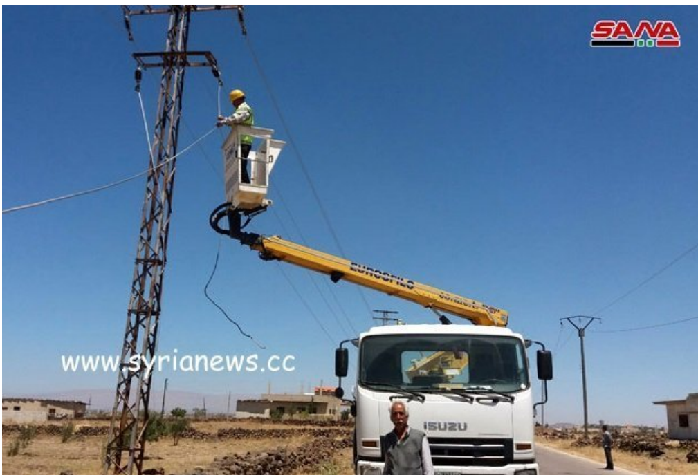
Syrian linemen re-electrify 30 towns in Quneitra.
