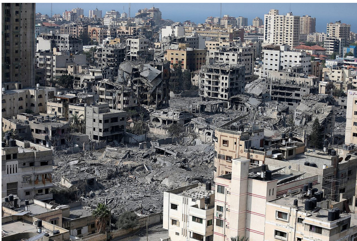
Devastation is seen in the area of Al-Rimal at the heart of Gaza City after Israeli bombing, October 23, 2023. (Mohammed Zaanoun/Activestills)
