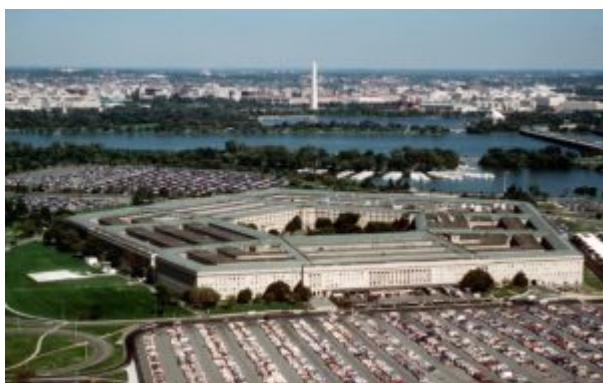
The Pentagon, headquarters of the U.S. Defense Department, as viewed with the Potomac River and Washington, D.C., in the background. (Defense Department photo)
