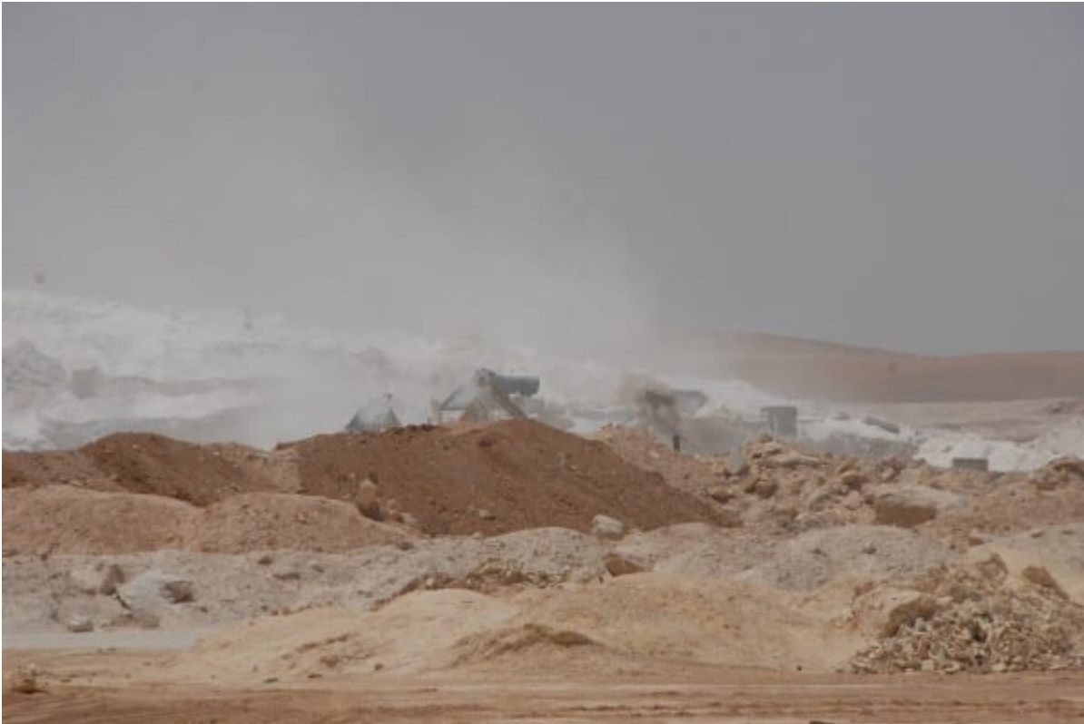
Building new road to Iraq...
