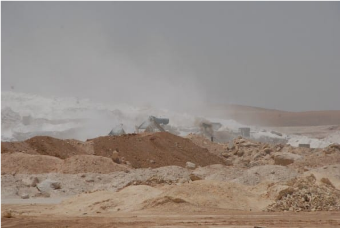
Building new road to Iraq...
