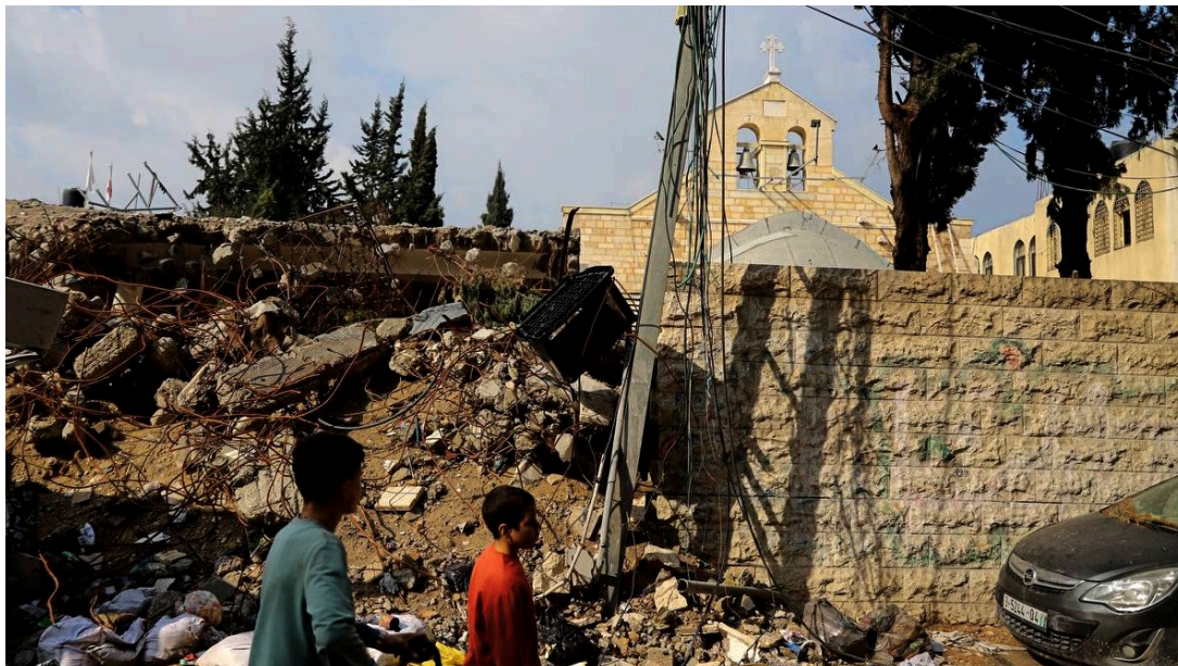
Gaza City's Greek Orthodox Church of Saint Porphyrius was damaged in Israeli bombardment, 2 January 2024 (Mohammed al-Hajjar/MEE)
