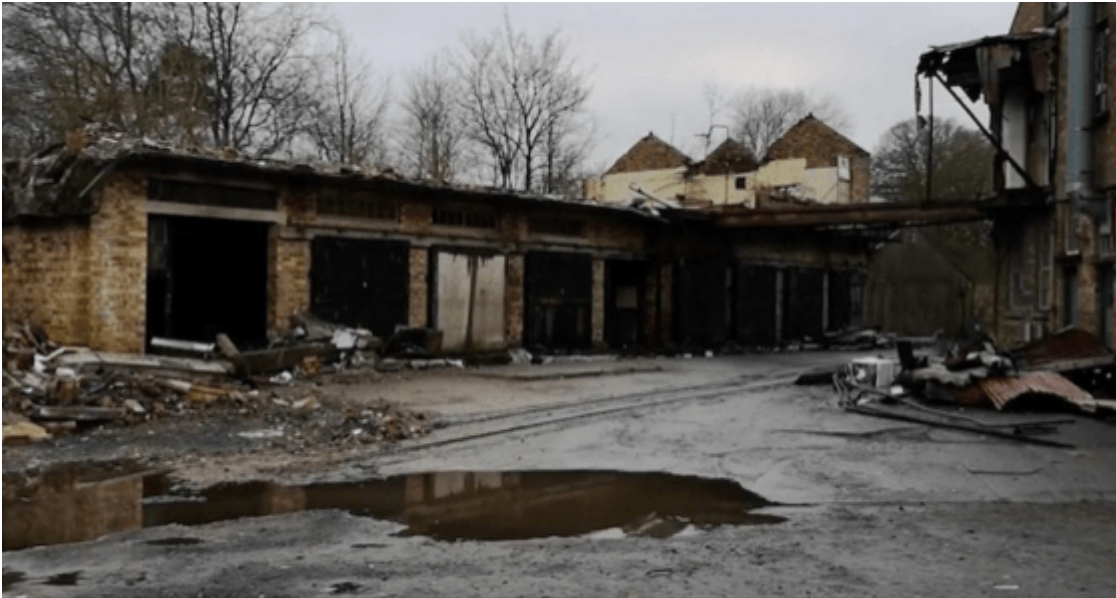
The partially demolished address at Gateside Mills. Photo: David Scott
