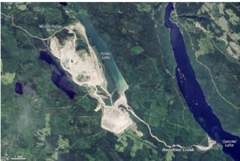
Before and after satellite photos of the Mount Polley copper mine area 2014. Note that in the lower photo the tailings lagoon is empty, the 6 foot wide Hazelton Creek is visible from space, the freshly-poisoned Polley Lake is no longer dark blue and there is floating debris in Quesnel Lake that is visible from space!
