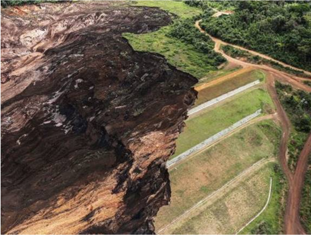
What's left of the upper section of the massive tailings lagoon after it liquified and collapsed
