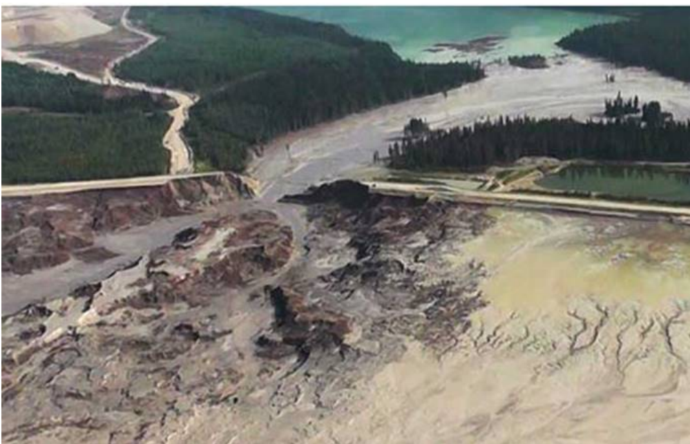
Aerial view of the 100 foot-tall earthen dam-wall of the Mount Polley gold and copper mine tailings lagoon after it dissolved in 2014 and spewed highly toxic sludge into Lake Quesnel, a world-famous
