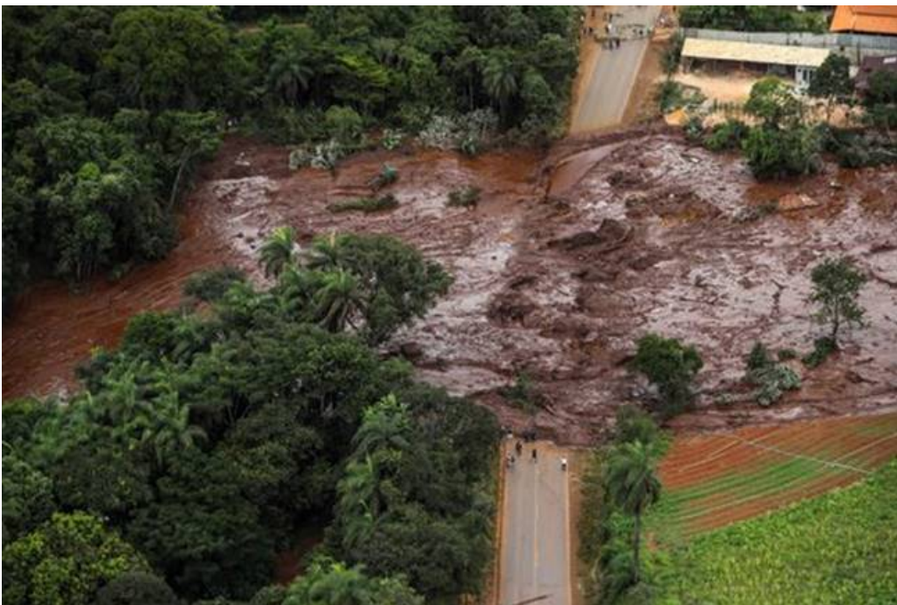
Toxic sludge overflowing a highway farther downstream. Note the damaged farm field (lower right)
