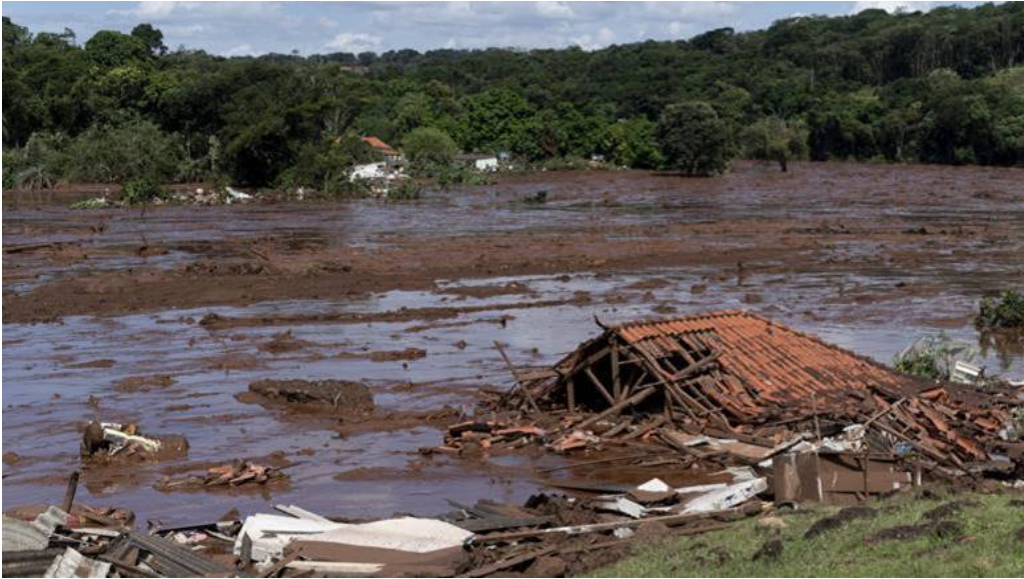
A sludge-demolished river-town home lies in ruins after the dam failure
