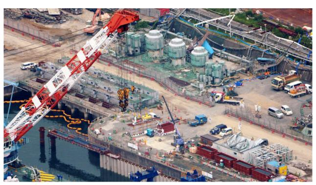
An aerial view shows workers wearing protective suits and masks work at a construction site (C) of the shore barrier to stop radioactive water from leaking into the sea at Fukushima Daiichi nuclear power plant on August 9, 2013. (Reuters/Kyodo)
