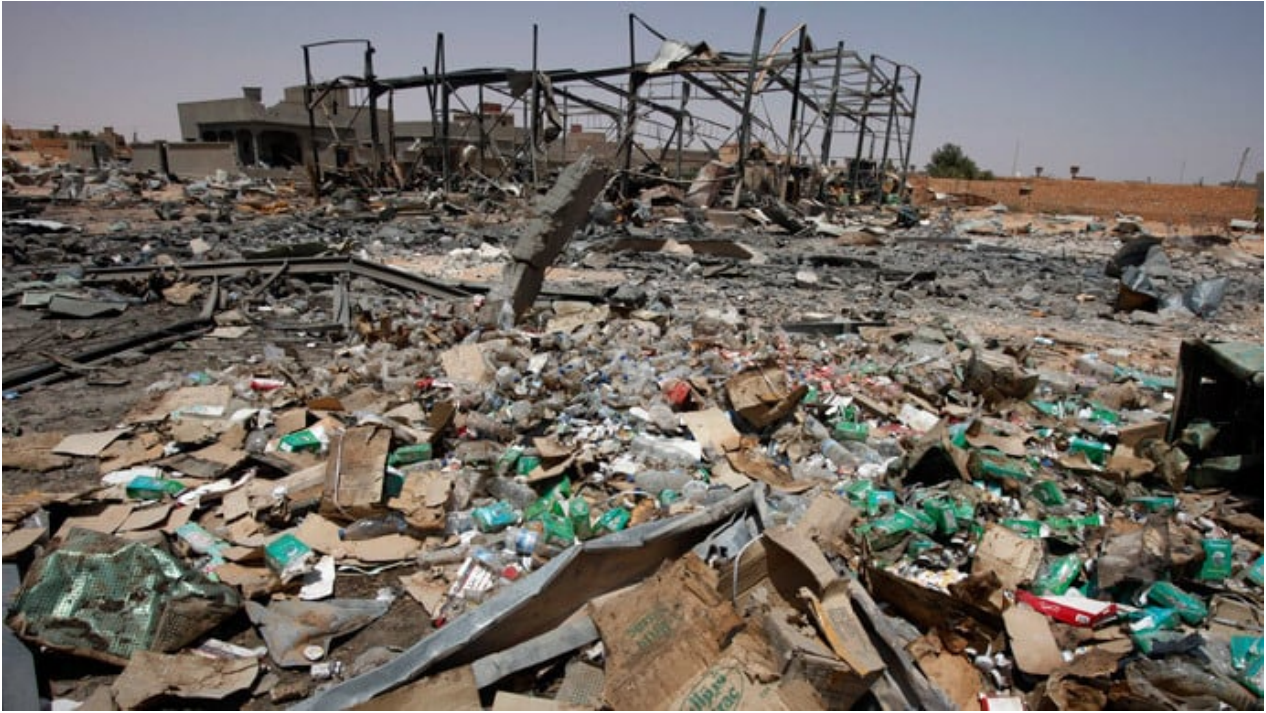
Image: A building used by Gaddafi troops to service vehicles is seen in rubble following a NATO airstrike in the town of Bir al-Ghanam in western Libya, August 8, 2011.(Reuters / Bob Strong)
