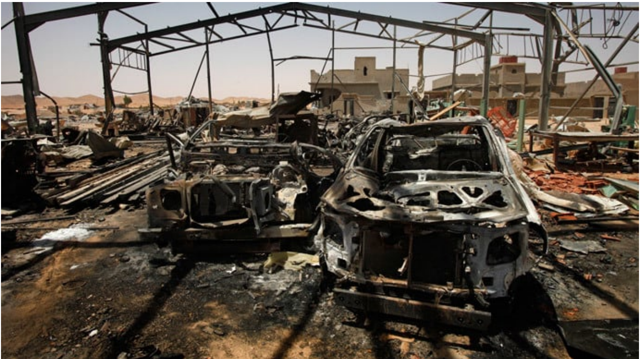
Image: A building used by Gaddafi troops to service vehicles is seen in rubble following a NATO airstrike in the town of Bir al-Ghanam in western Libya, August 8, 2011.(Reuters / Bob Strong)
