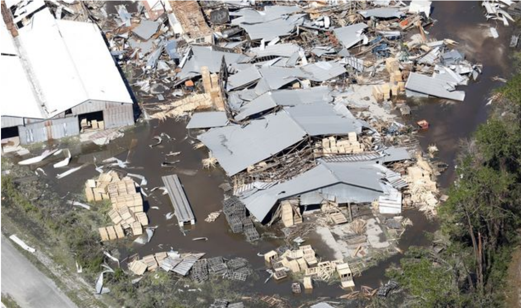
Damage from Hurricane Michael (Source: US Defense Department)
