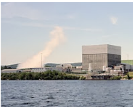
Vermont's Nuclear Plant
