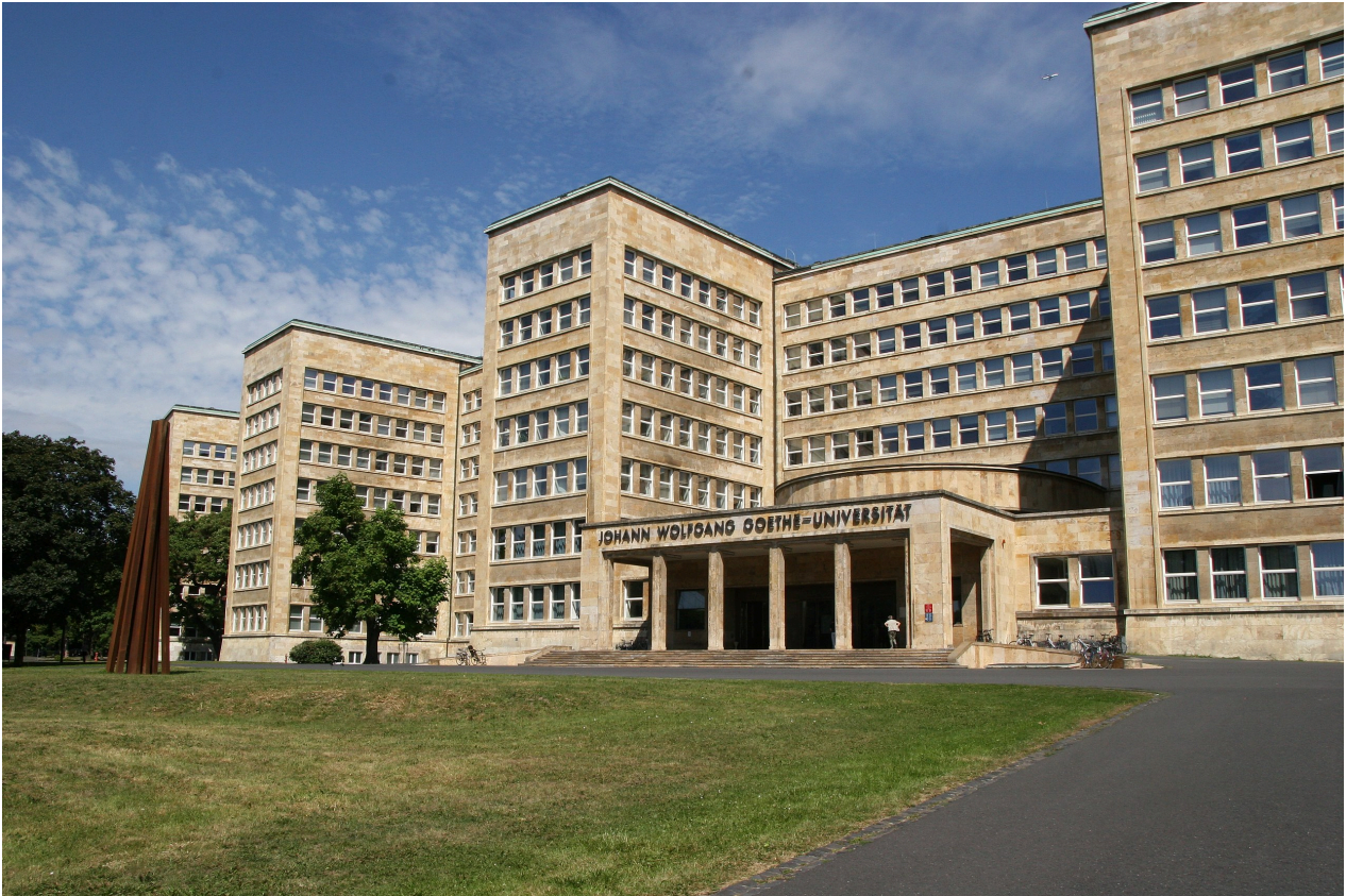
IG Farben Building, Frankfurt, completed in 1931 and seized by the Allies in 1945 as the headquarters of the Supreme Allied Command. In 2001 it became part of the University of Frankfurt. (Licensed under CC BY-SA 3.0)
